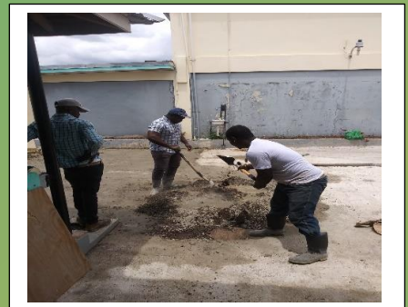
Dumpling and his team busy mixing cement.
